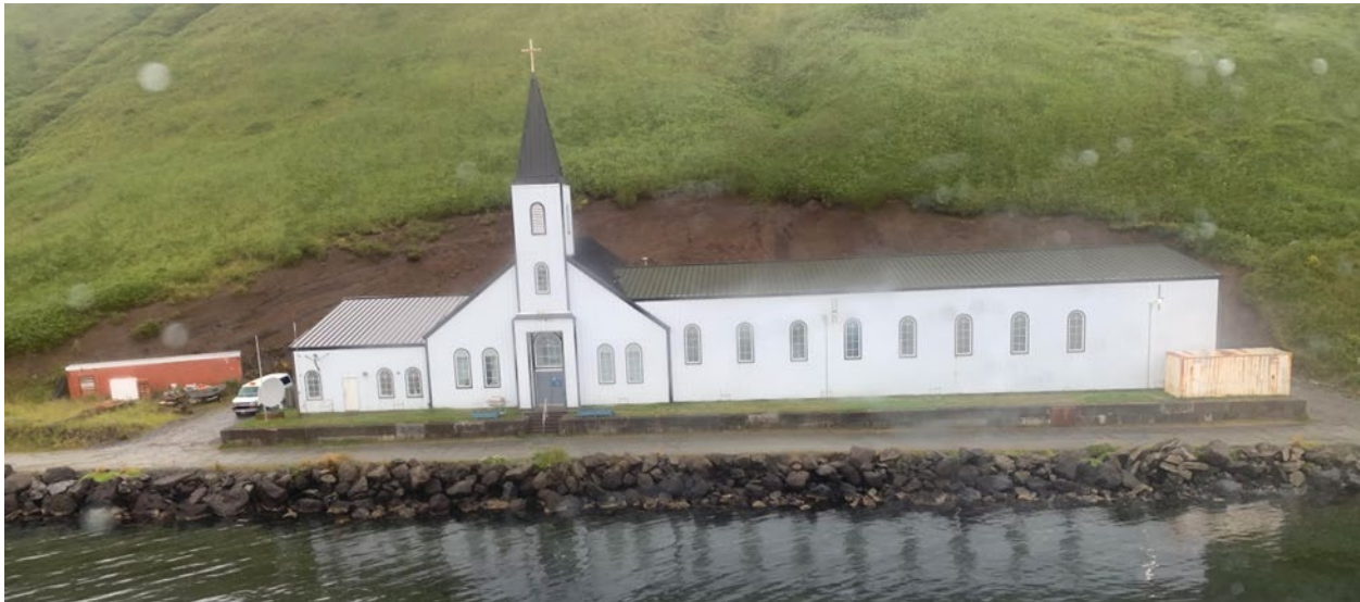
Plate 6. Safe Harbor Church/Community Building
