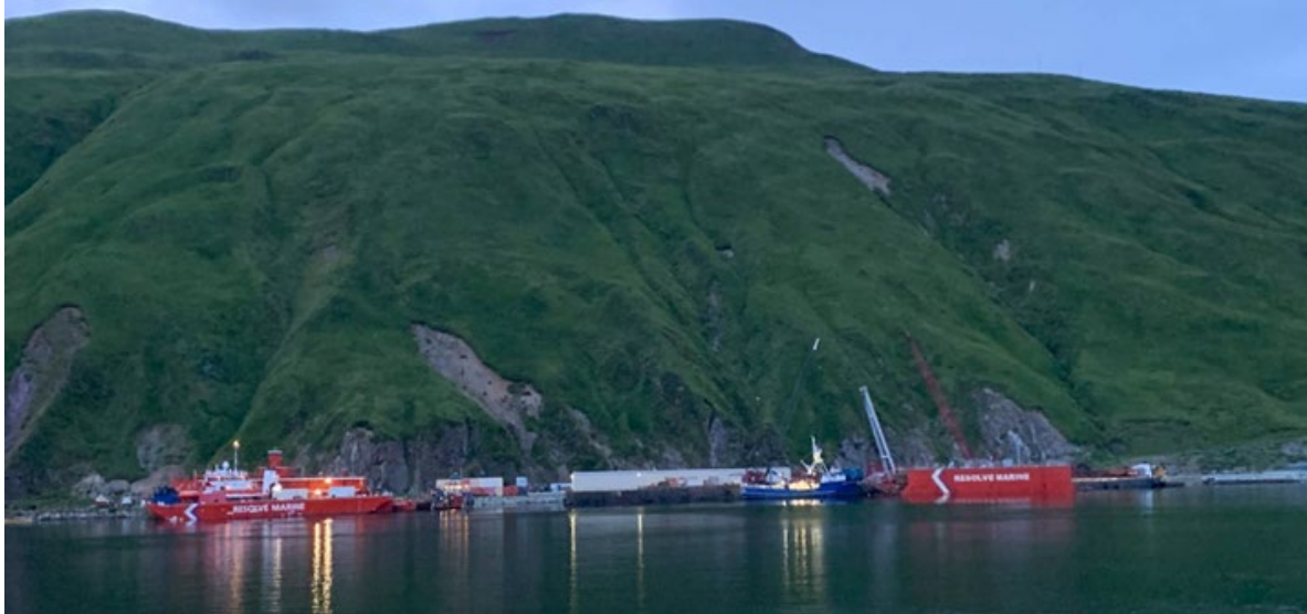
Plate 15. Resolve Marine Unalaska Facilities
