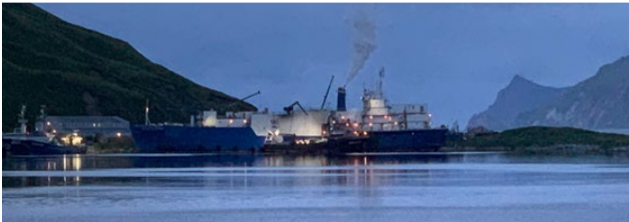
Plate 13. Northern Victor Processing Facility
