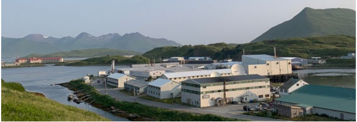
Plate 11. Alyeska Processing Complex
