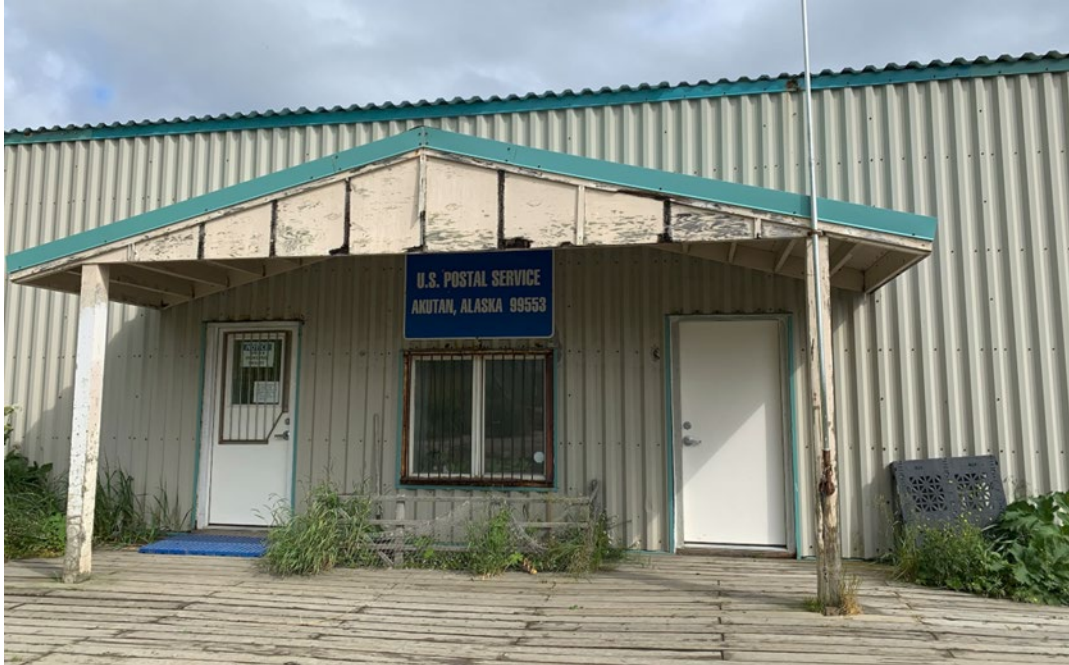
Plate 8. Akutan Post Office
