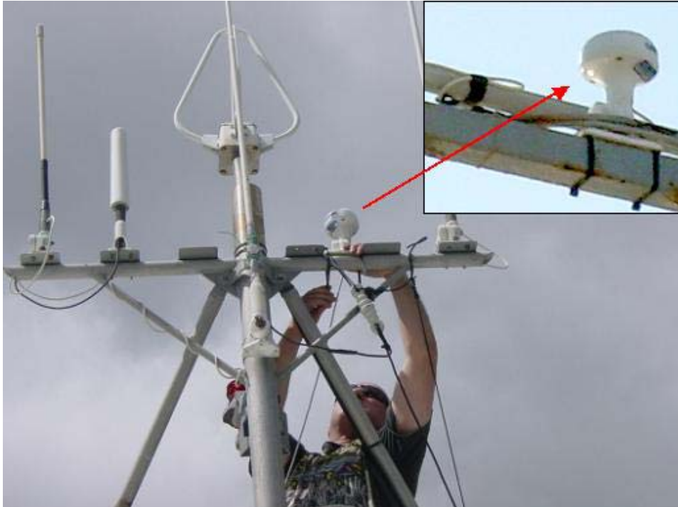
Figure A3. GPS receiver installed in the rigging of a vessel and a close up photograph of the mounted GPS.
